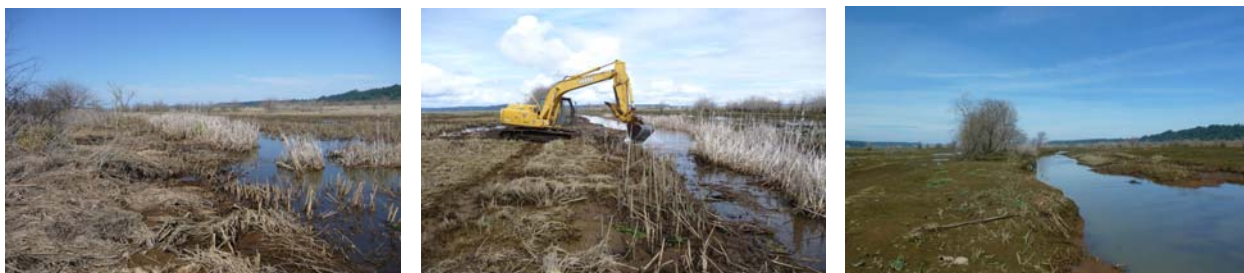
FIGURE 16. PHOTOGRAPHS OF LESCHI SLOUGH BEFORE, DURING, AND AFTER DREDGING
